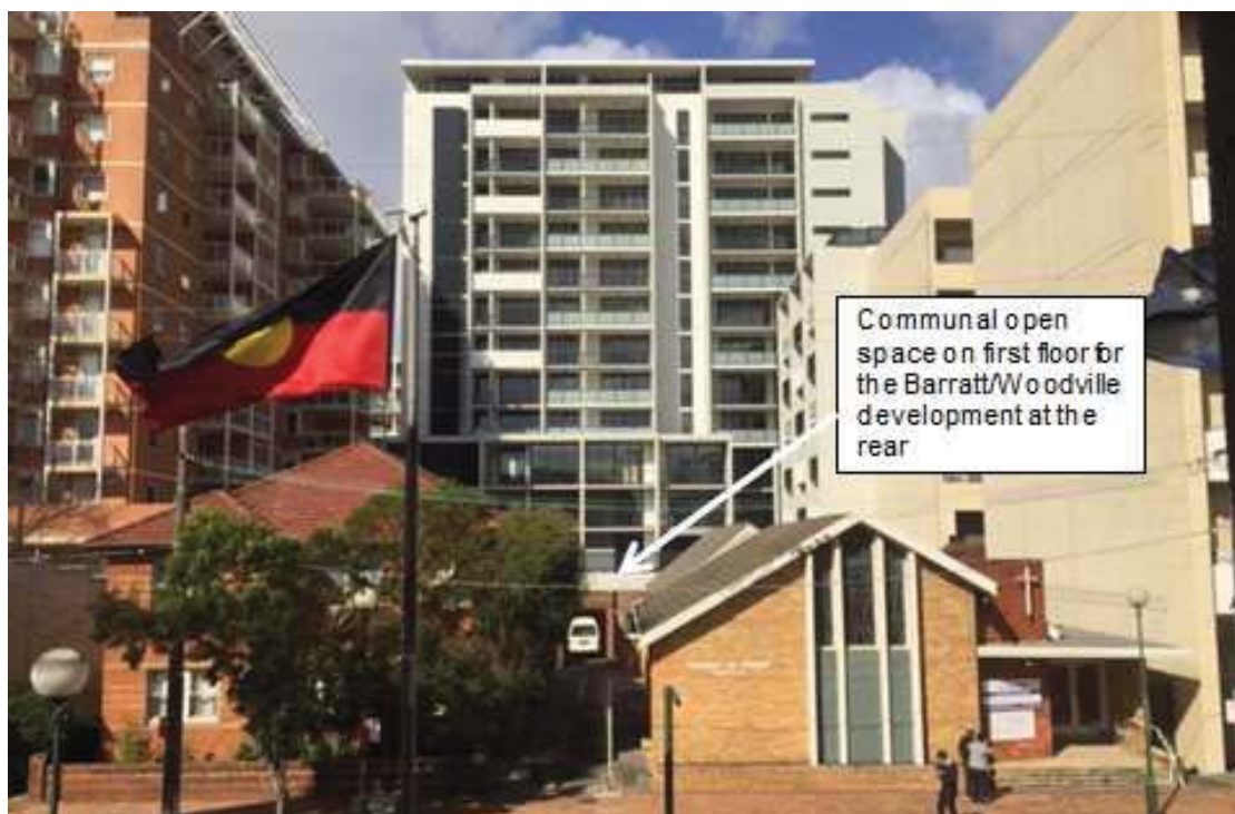
Figure 4: First floor Communal Open Space at the rear of Barratt/Woodville building
