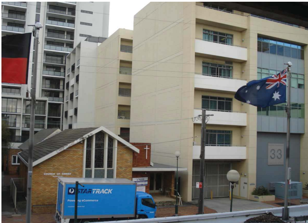
Figure 3: Six storey commercial building to the west of Subject Site
